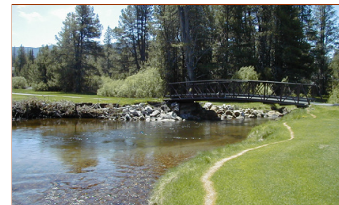
Several undersized bridges along this reach are located within the floodplain, constricting flow and accelerating velocities leading to erosion downstream.
