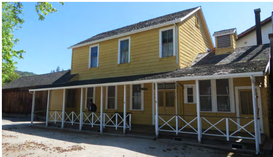
Figure 15. The Kitchen Annex is located behind the Hotel and oriented perpendicular to street along the side property line with the Barracks Building (photo: Garavaglia Architecture, Inc., April 2013).
