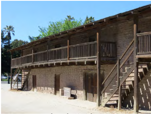
Figure A66. Southern half of the east elevation, looking southwest.
