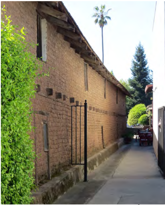
Figure A70. West elevation, looking southeast.
