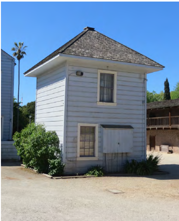
Figure A58. North elevation.
