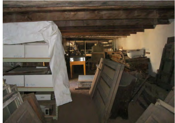
Figure A75. Ground level storage, looking south.
