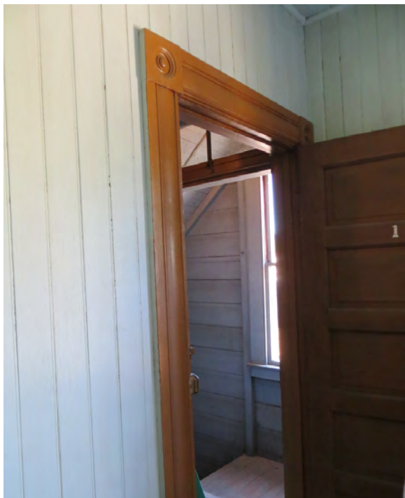
Figure A38. Second floor rooms as bulls-eye molding and 5-panel doors, like those found in the Hotel Annex.
