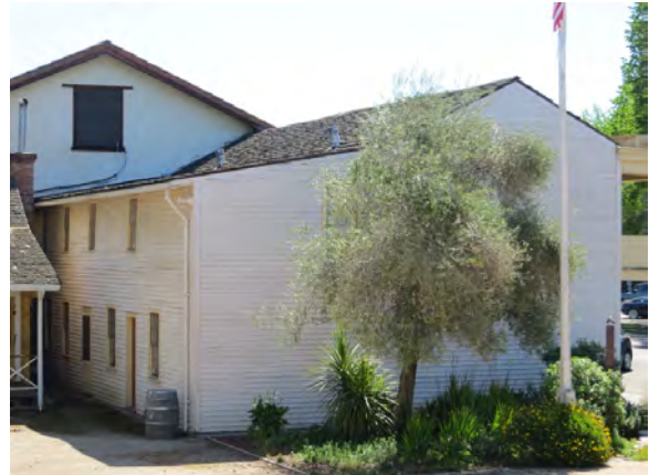
Figure A2. West and north elevations.
