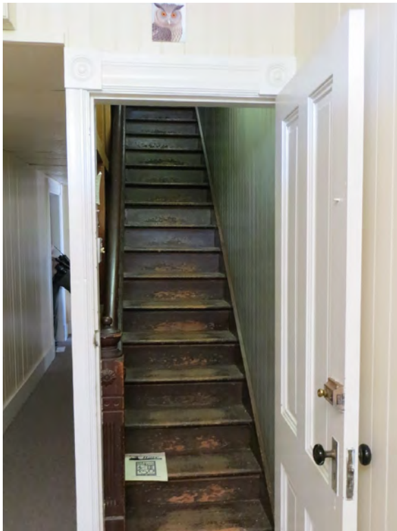
Figure A52. The original stair has been enclosed to satisfy safety codes.
