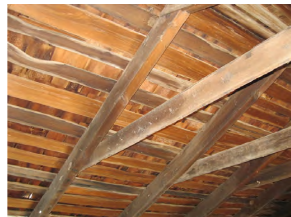
Figure A79. Roof framing, sheathing, and shingles as viewed from below.
