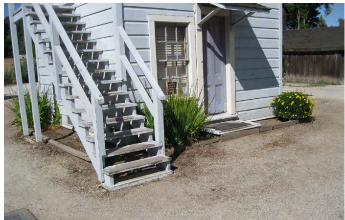
Figure 55. This image of the Tank House illustrates the common threshold issues when considering universal access. Most entry points are 1-2 steps above grade.
