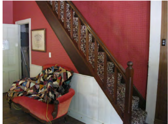
Figure A12. Detail of the eastern stair. Mechanical equipment is in the under-stair closet.
