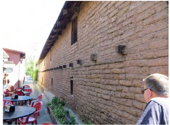
Figure A67. West elevation, looking northeast.
