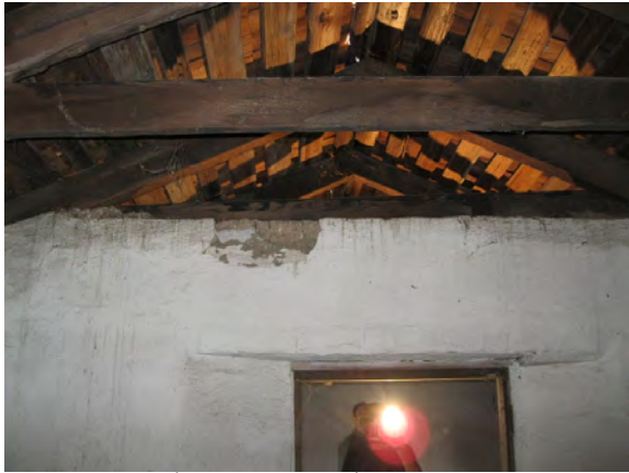
Figure A82. This cross wall has no fill material.
