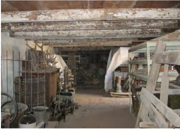
Figure A74. Ground level storage, looking north.
