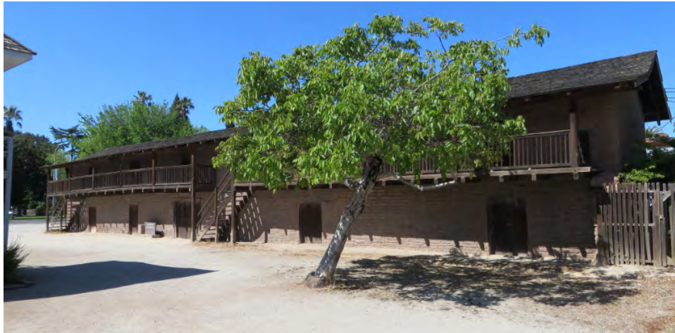
Figure 18. The east elevation of the Servants' Quarters as viewed from the rear of the park site (photo: Garavaglia Architecture, Inc., April 2013).
