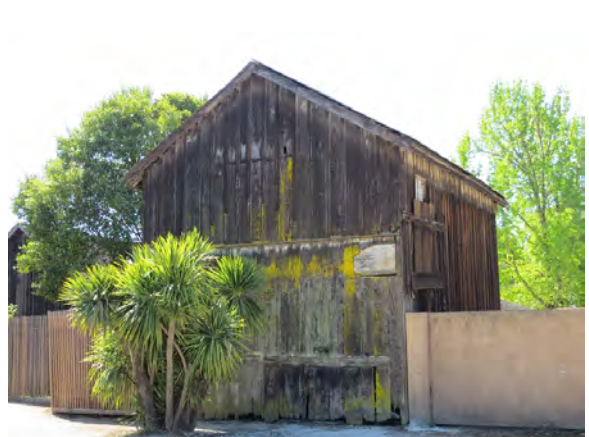
Figure A88. North elevation.
