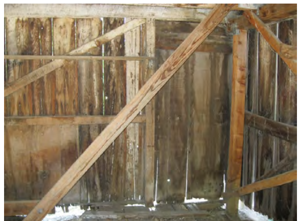
Figure A90. Interior detail showing a former door opening.
