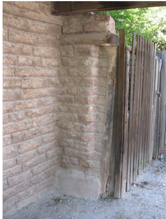
Figure A72. Detail of the northeast corner under the balcony.
