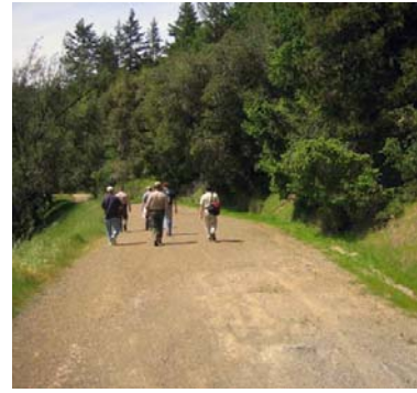
Access road below road wash-out.
