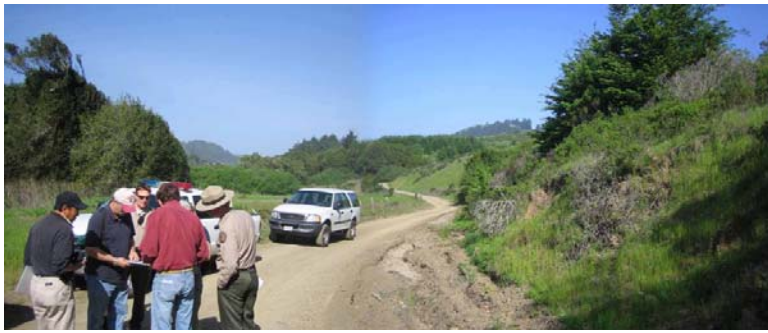
Site A - looking west - eroded roadway swale on left.
