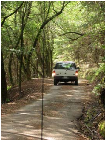
Narrow entry from residential area.
