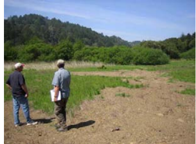
Site A - looking southwest at eroded area.
