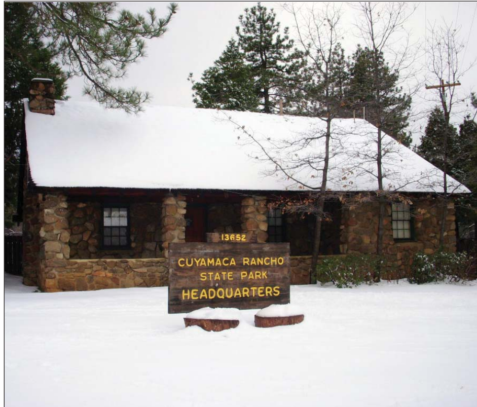
Park Headquarters Building
