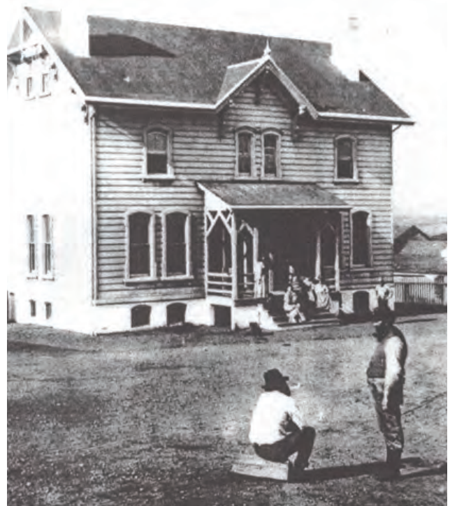
Keepers House at Pigeon Point in 1873 (source: Ann Steel's Collection)
