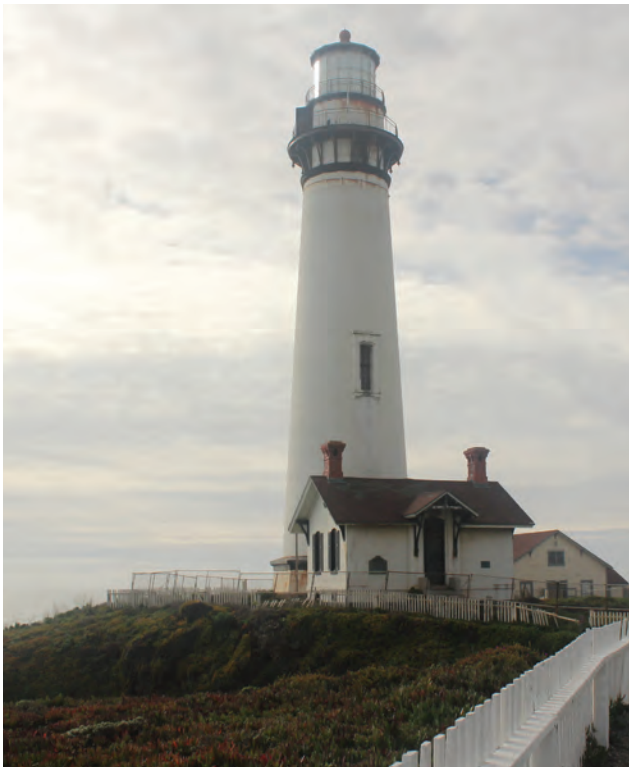
Lighthouse and Attached Oil House
