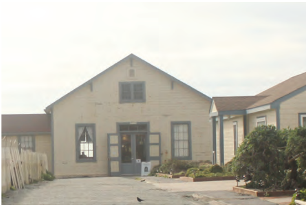
Fog Signal Building (east facade)
