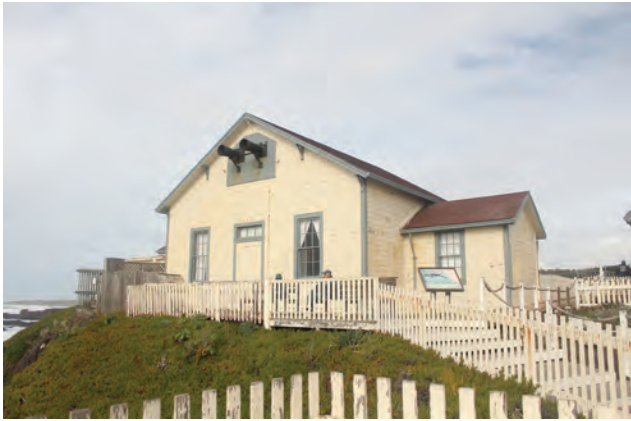
Fog Signal Building (west facade and deck)
