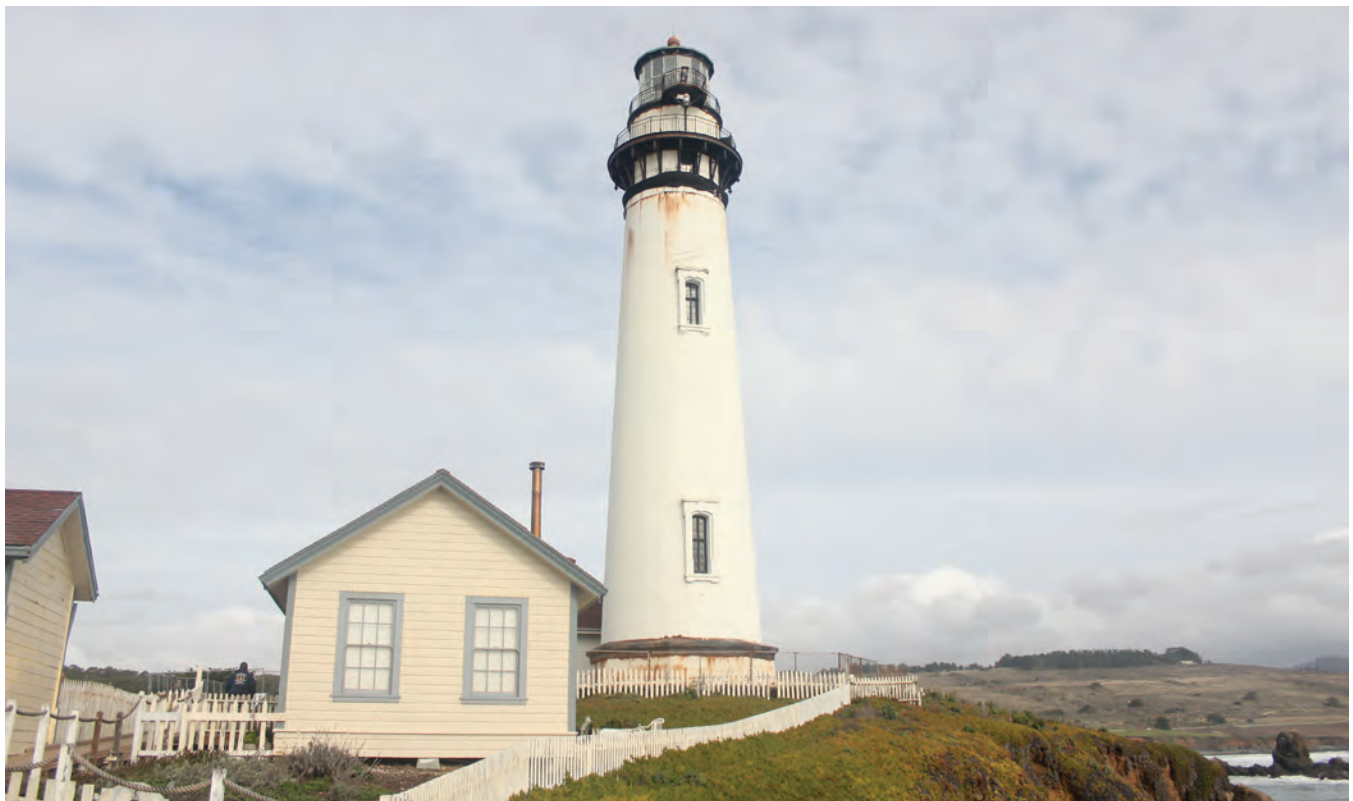
View of Lighthouse and Carpenters Shop from Deck
