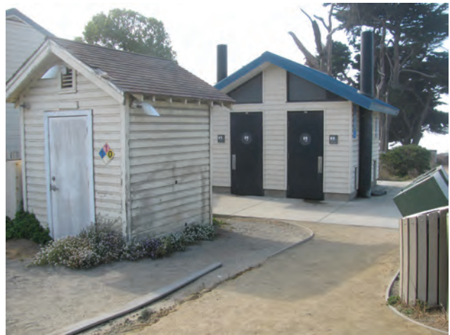
Decomposed Granite in front of Restroom
