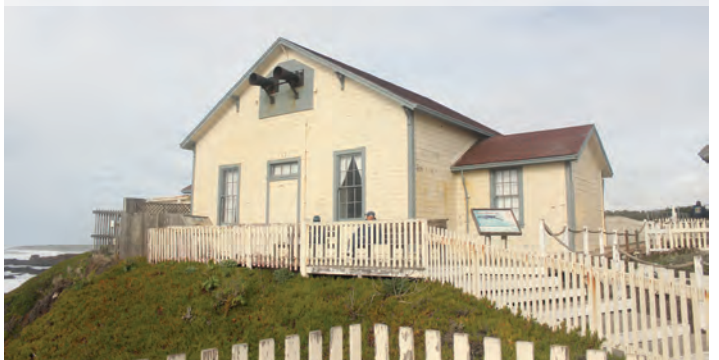
deck on Fog Signal Building
