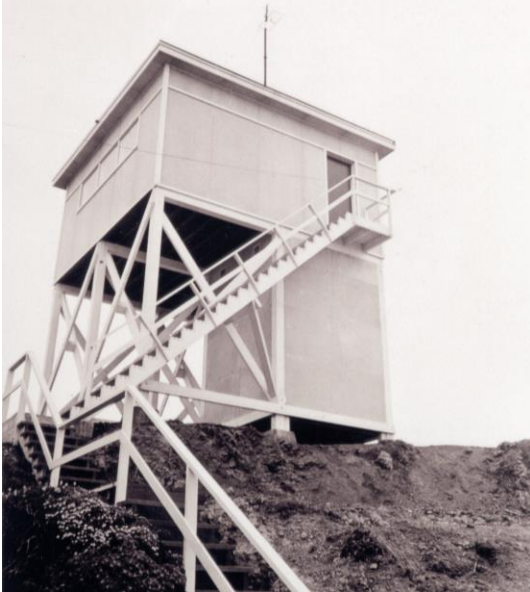
RAadar BeaCON (RACON) Tower on Moro Rock.
