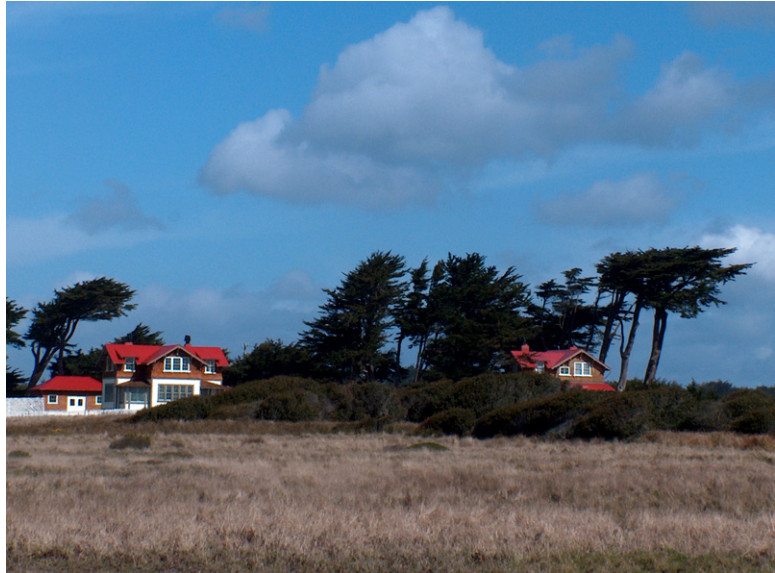
Rehabilitated Principal and First Assistant Lightkeepers' houses, from left to right, as viewed from the preserve
