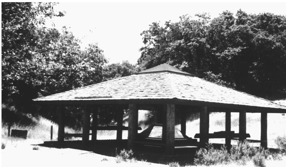
Interpretive Shelter at Partridge Farm
