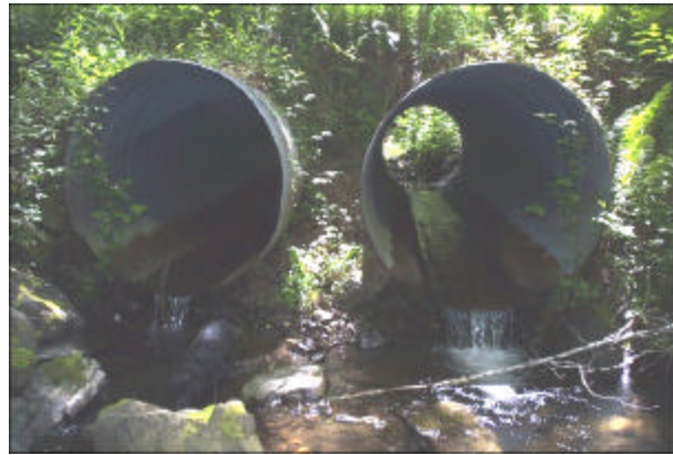
Double-barrel culvert on West Branch of East Fork Mill Creek.
