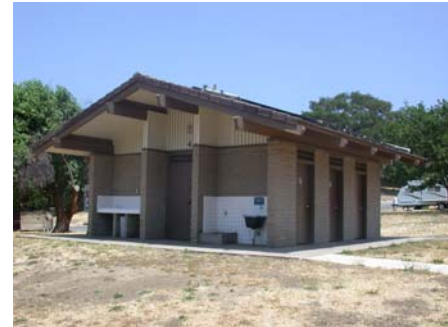
Restroom facilities at the main campground
