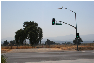
Existing signal on Branham Lane
