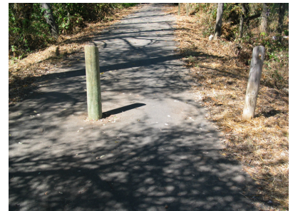
Movable bollards in road restrict vehicular access
