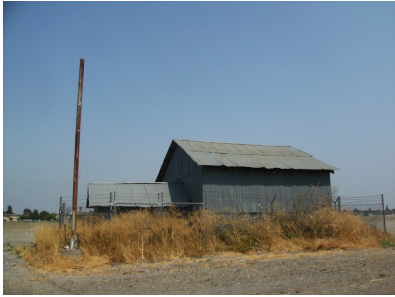
Existing pump house
