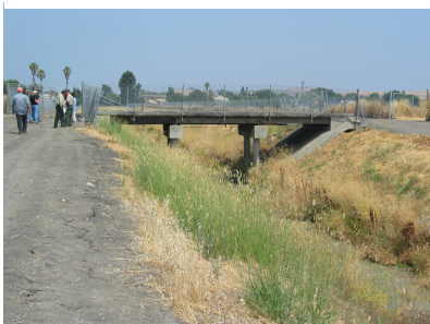
Bridge over Canoas Creek channel
