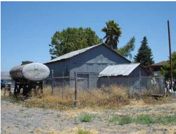
Well pump house
