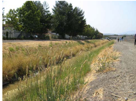
Canoas Creek drainage channel
