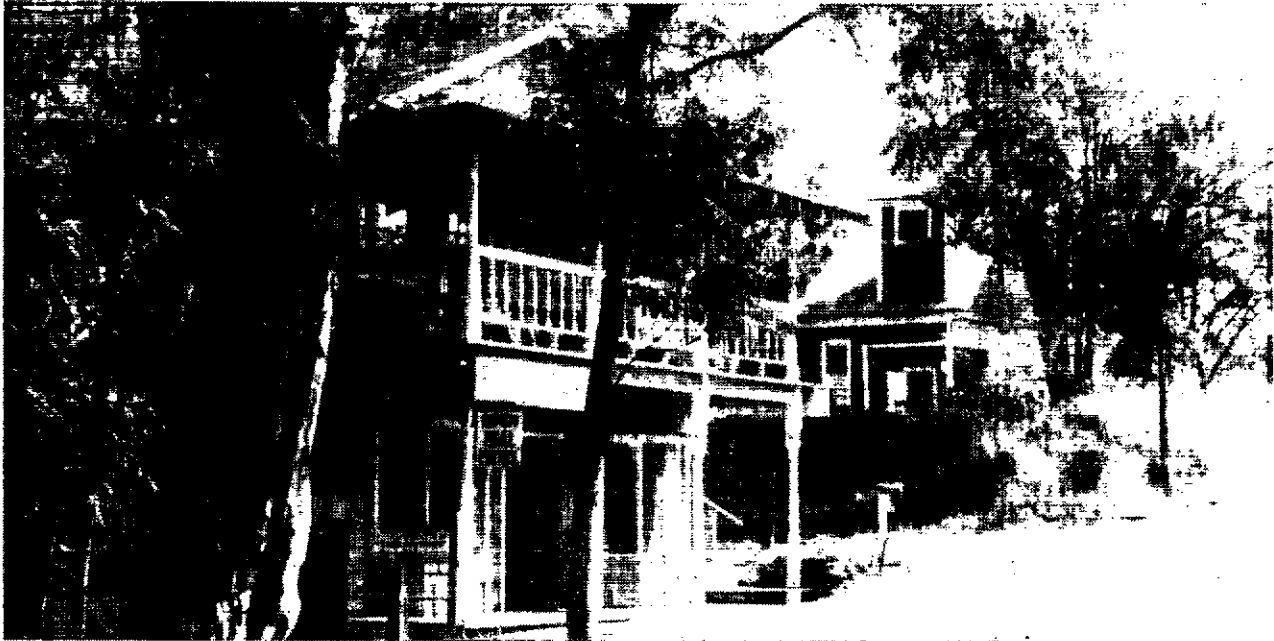
Antique shop located in old schoolhouse and realty office are two commercial businesses recently acquired
