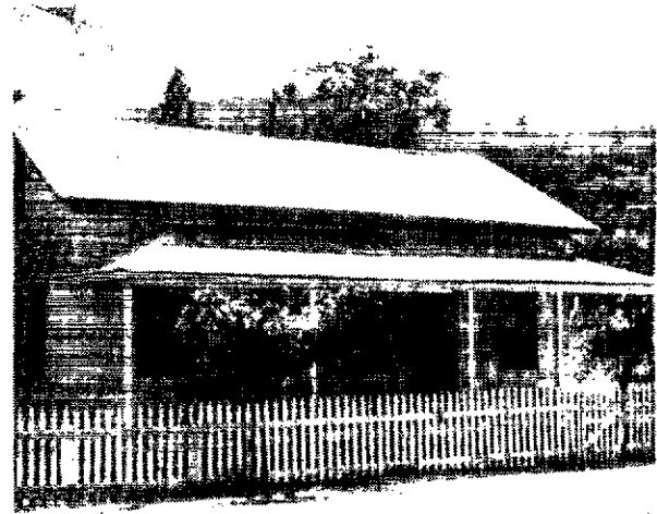
Weller House - originally constructed in 1852, proposed for restoration as a house museum
