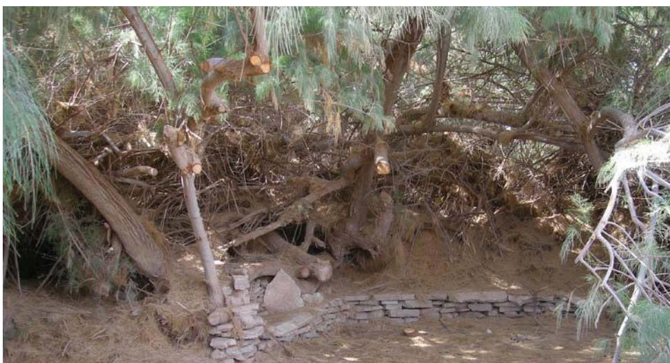
Stone retaining wall.
