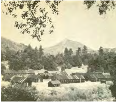
CCC camp buildings in Green Valley with Stonewall Peak in the background ca. 1934
