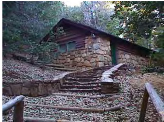
North KYBO building at the former Camp Hual-Cu-Cuish prior to the Cedar Fire ca. 1990's
