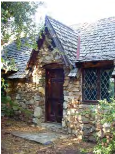
Front door of former Mack Ranch House November 2013
