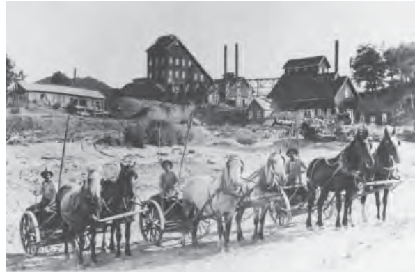
Scrapers moving mine tailings at Stonewall Mine ca. 1895
