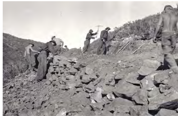
CCC crewmen constructing trail with picks and shovels September 1934
