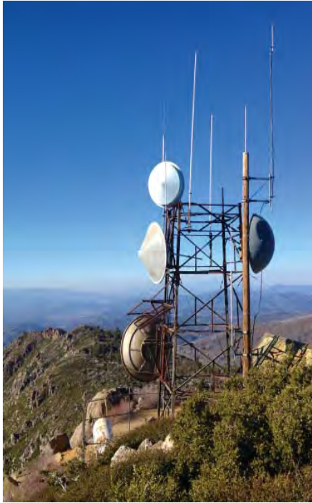
Communications tower on Cuyamaca Peak February 2014
