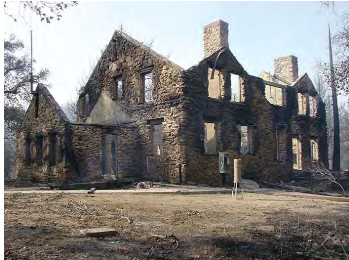
The Ralph M. Dyar House and former Park headquarters after the Cedar Fire
