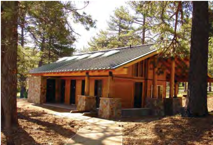
Combination shower and restroom building at Los Vaqueros Equestrian Group Campground January 2013
