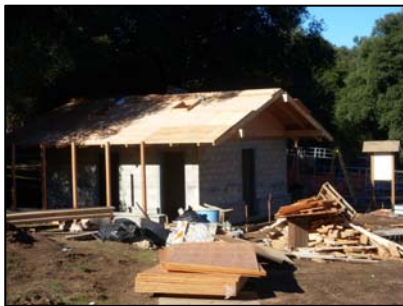
Remodeled Restroom/Shower Building at Green Valley Horse Camp
