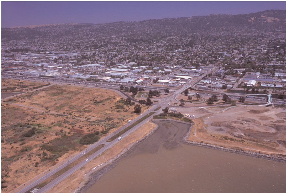
Berkeley lands with I-80, University Avenue interchange & pedestrian overpass
