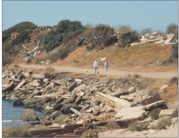
Concrete debris along the Albany Neck
