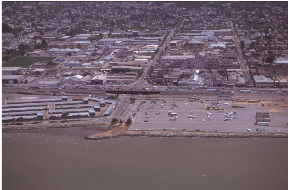
Golden Gate Fields parking and stable at foot of Gilman Street
