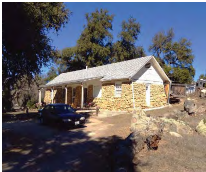
Merigan Ranch Stone Cabin at the southern end of CRSP August 2012
