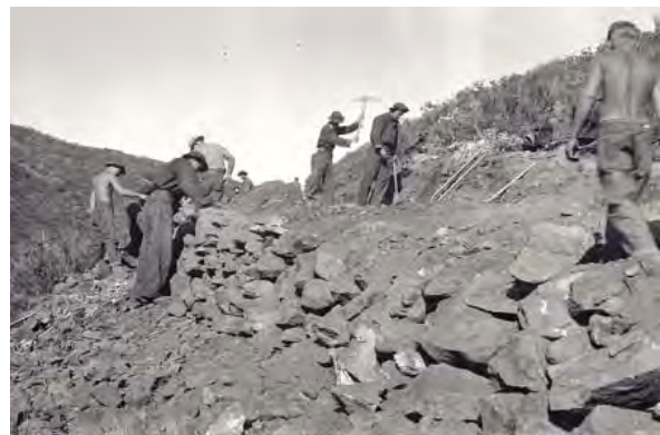
CCC crewmen constructing trail with picks and shovels September 1934
