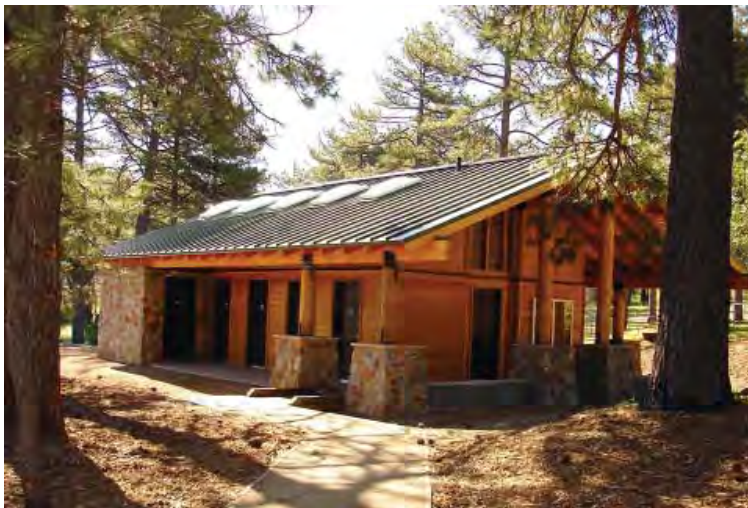
Combination shower and restroom building at Los Vaqueros Equestrian Group Campground January 2013
