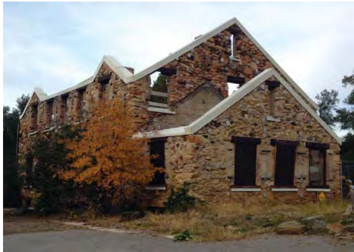
The Ralph Dyar House - post-Cedar Fire structural stabilization completed September 2013
