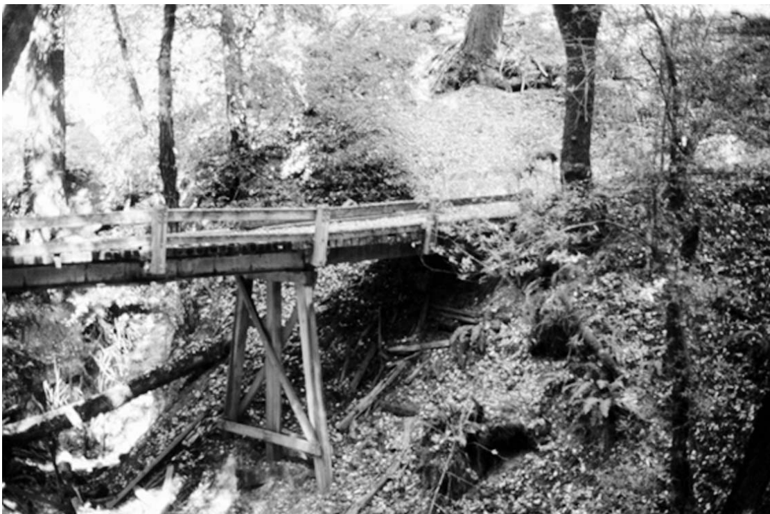
Bridge, Saratoga Toll Road
