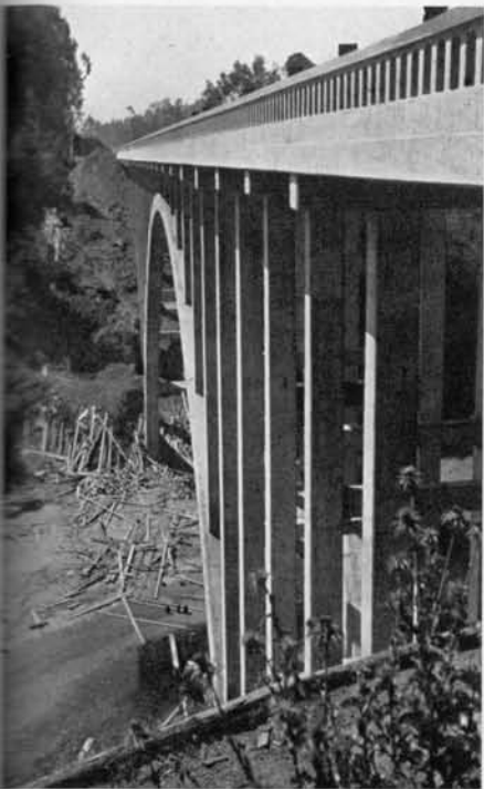
Russian Gulch Bridge, a graceful spandrel arch structure 526 feet, 9 inches long on the Mendocino Coast highway was dedicated June 9 when Secretary of State Paul Peek cut the ribbon. The old structure was a timber trestle built 30 years ago.
