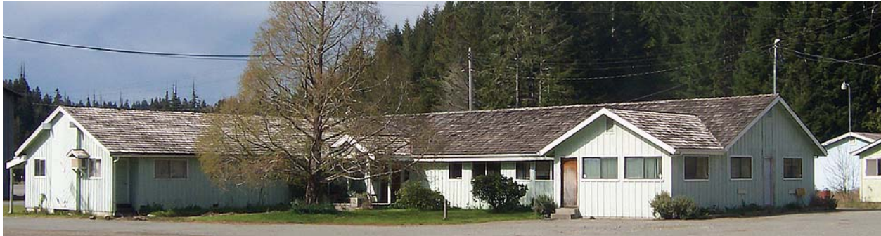
Office building at the former mill site, Source: EDAW 2008
