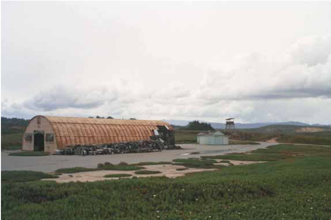
View of existing facilities near storage bunkers
