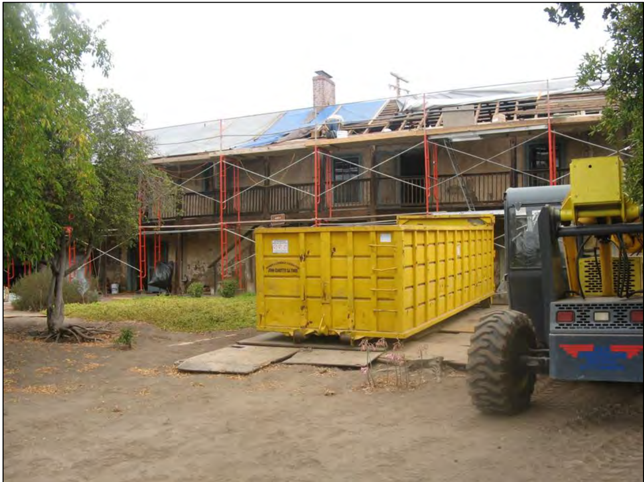
Image 9: Roof repair and seismic stabilization project at the Blue Wing Inn.
