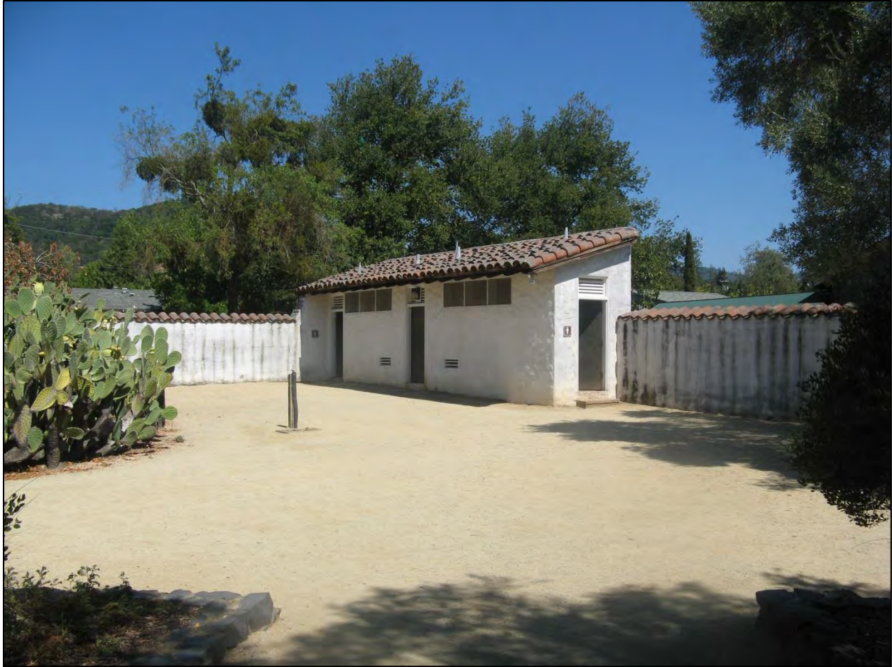
Image 44: Restroom facilities in the Mission Courtyard.
