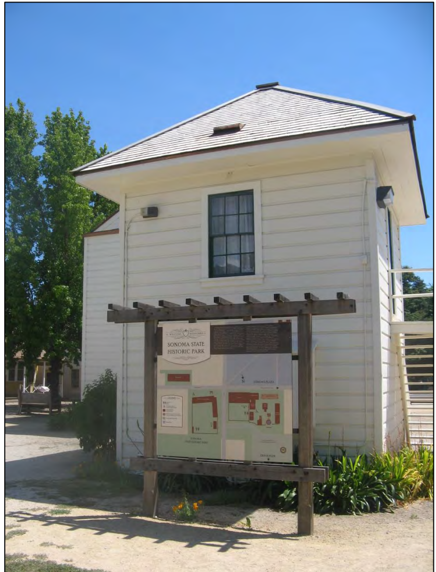
Image 37: Toscano Water Tank House.
