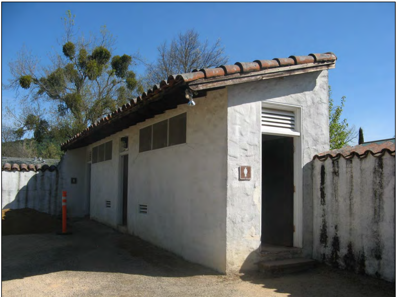
Image 8: Restroom facility in Mission San Francisco Solano Courtyard.
