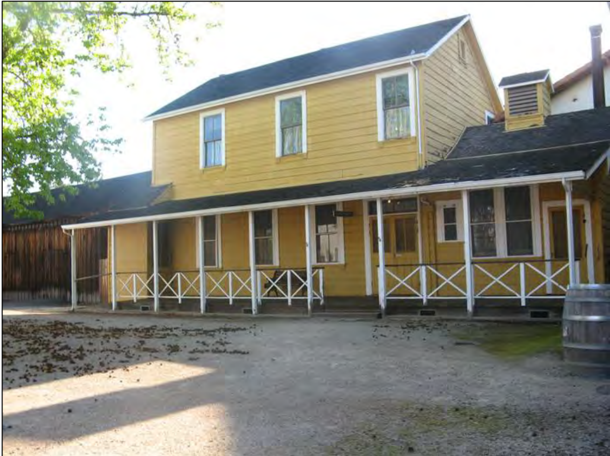
Image 34: Toscano Kitchen Annex.
