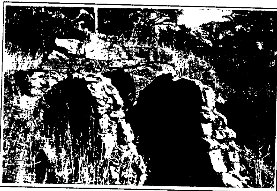
During the 1930's, the Civilian Conservation Corps constructed a number of culverts in the park.
