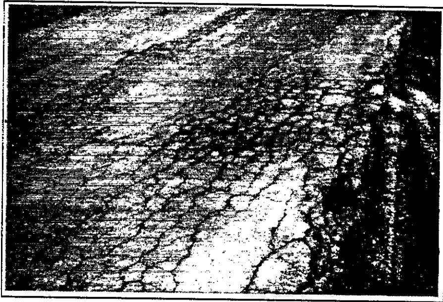
Park roads are minimally maintained and are deteriorating.
