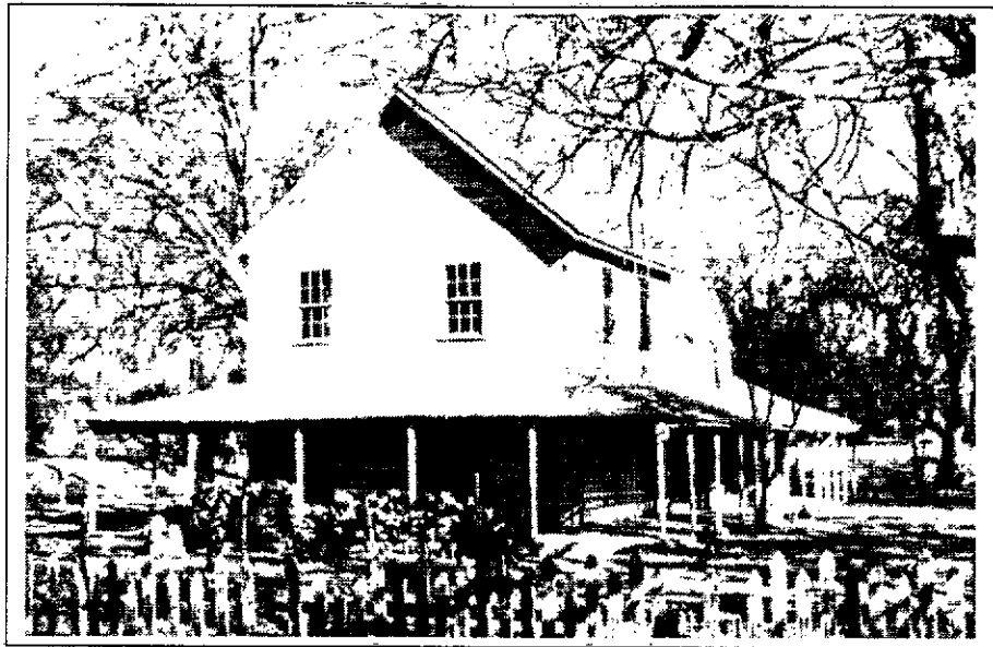
The Anderson Ranch house is associated with the early settlement of Lake County and the development of farming and ranching in the Clear Lake area.
