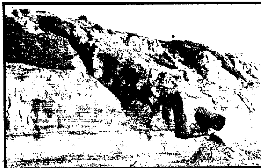
Bluff erosion was accelerated by the failure of a number of drain pipes.
