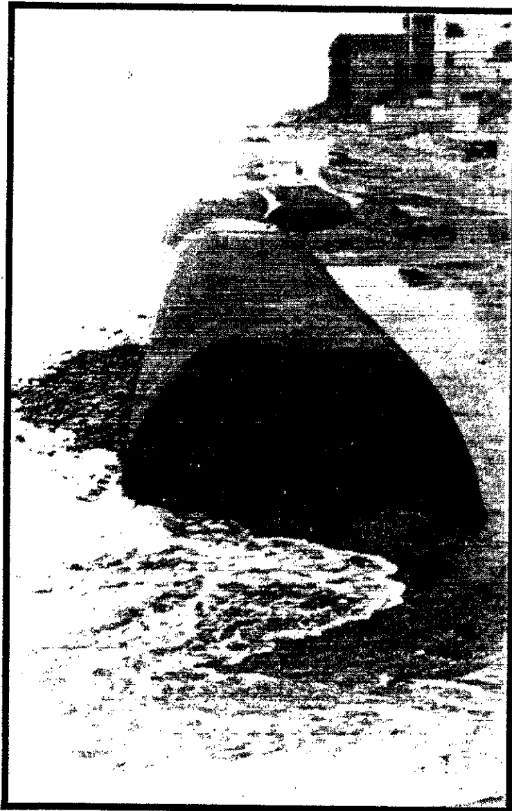
Beach protection devices, such as this Longuard tube, may be necessary to retain the beach in Area 2.
