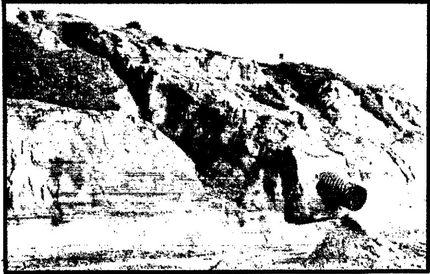
Bluff erosion was accelerated by the failure of a number of drain pipes.
