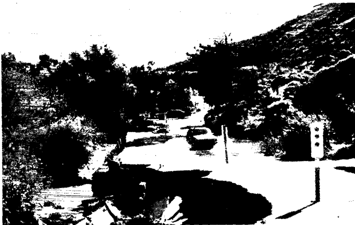
Heavy rainfall in the spring of 1978 resulted in extensive flooding in the lower Gaviota Creek floodplain and severe erosion at the ford on the county-owned access road.
