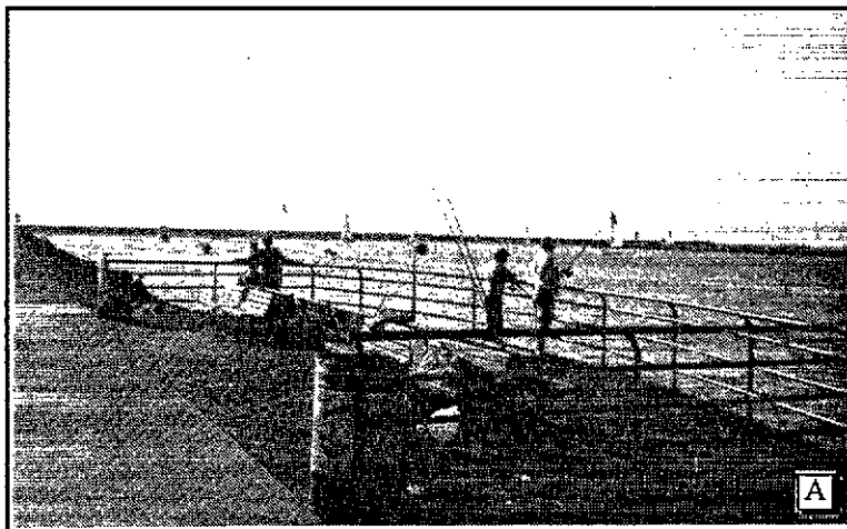
Plate 10 Fishing and View Piers (Marina del Rey)
