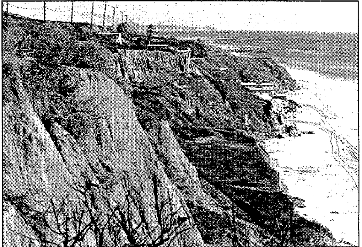
Eroding coastal terrace. Note the charred vegetation from Green Meadows Fire (1993).
