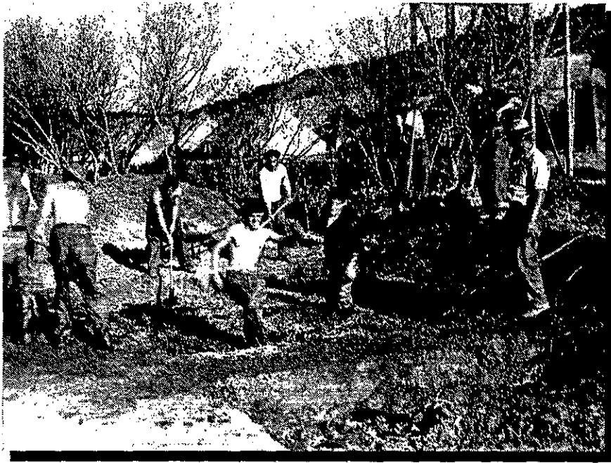
The old time adobedero made his bricks by an ancient method copied here by the restoration crew. The mud and straw were mixed in pits. The adobe was then moulded in a wooden frame and allowed to dry in the hot sun.
