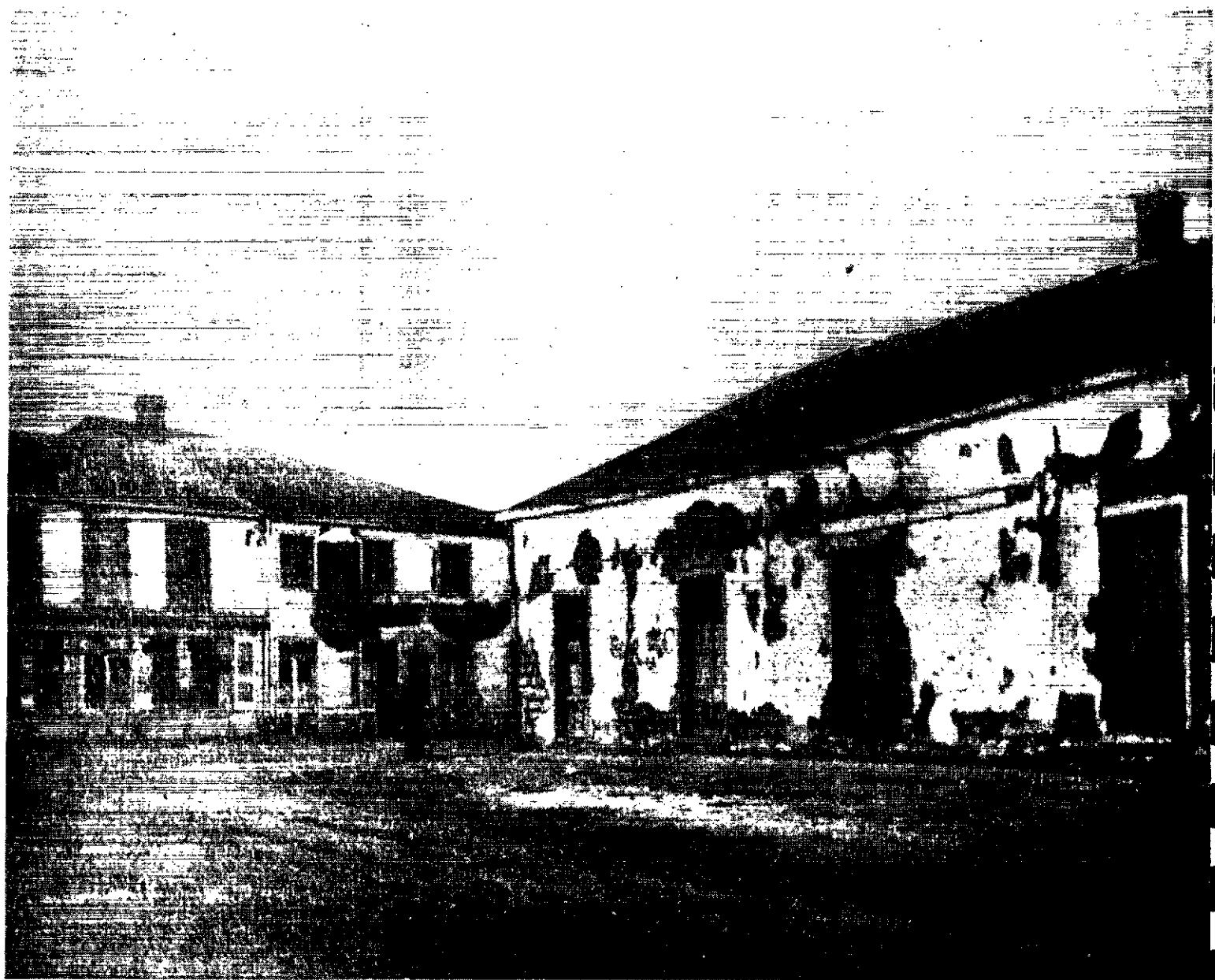
Adobe, formerly at corner of Pearl and Tyler
