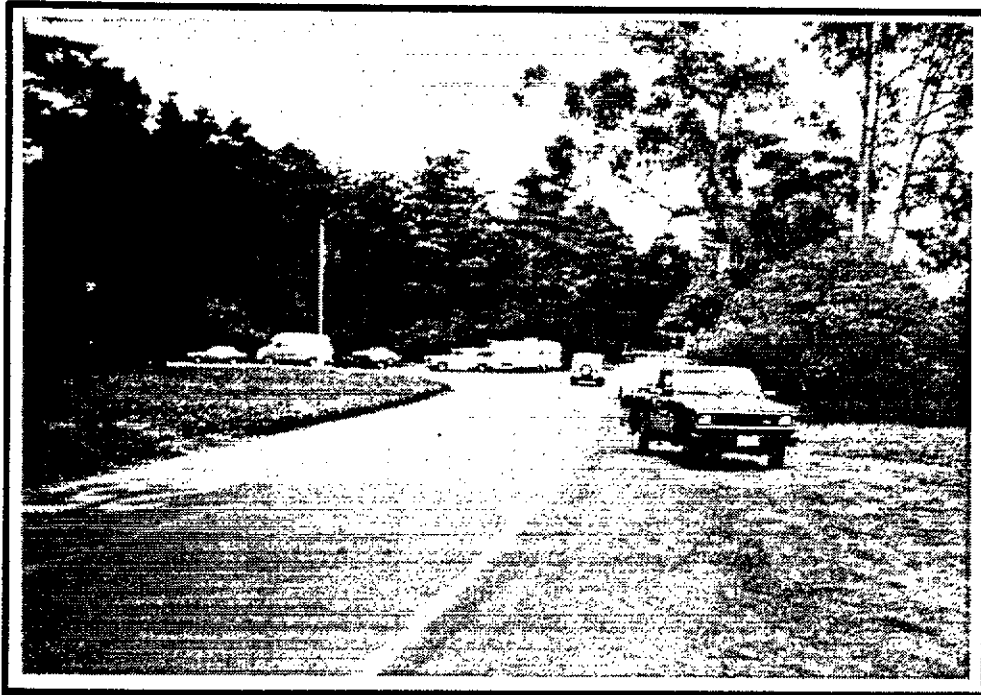
Lower State Park Road at campground entrance
