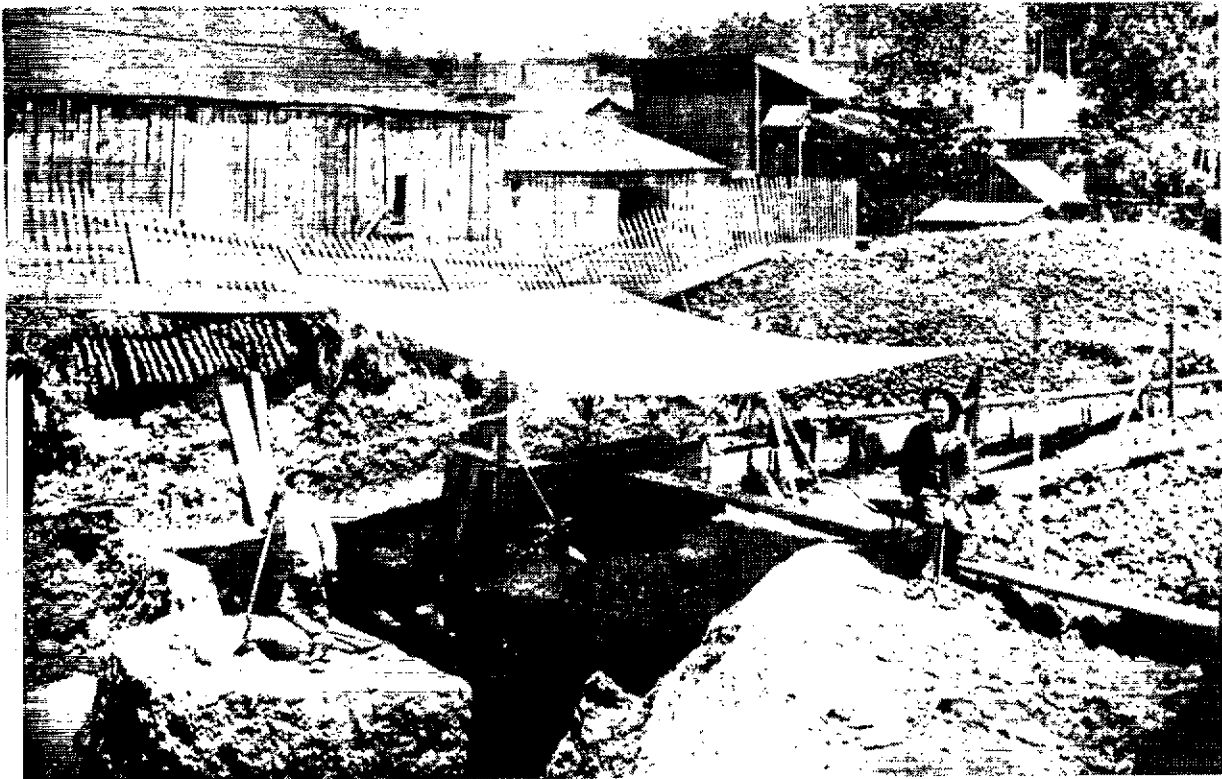
Mining activities within the town during a late mining frenzy undermined many buildings. Such sites will be preserved.
