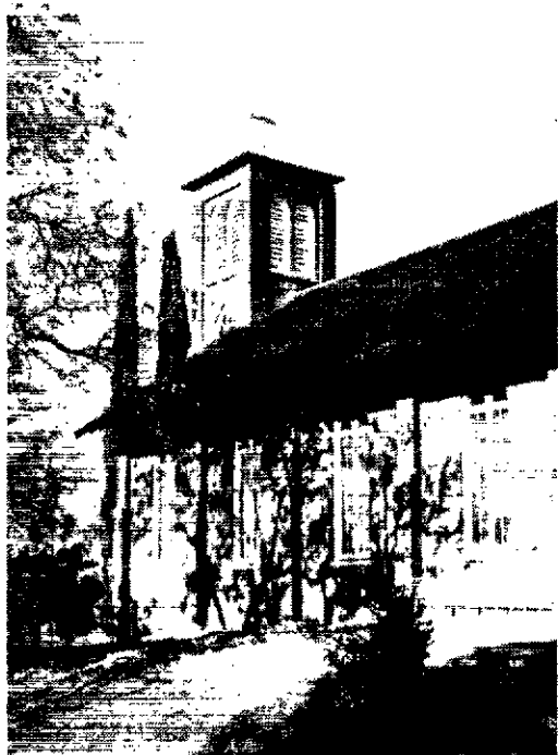
St. Anne's Catholic Church is slated for early restoration.
