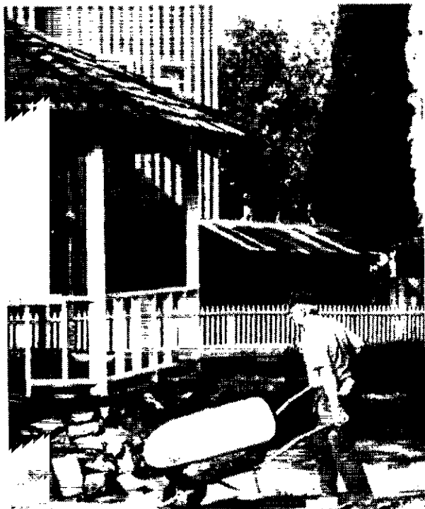
Park maintenance in progress
