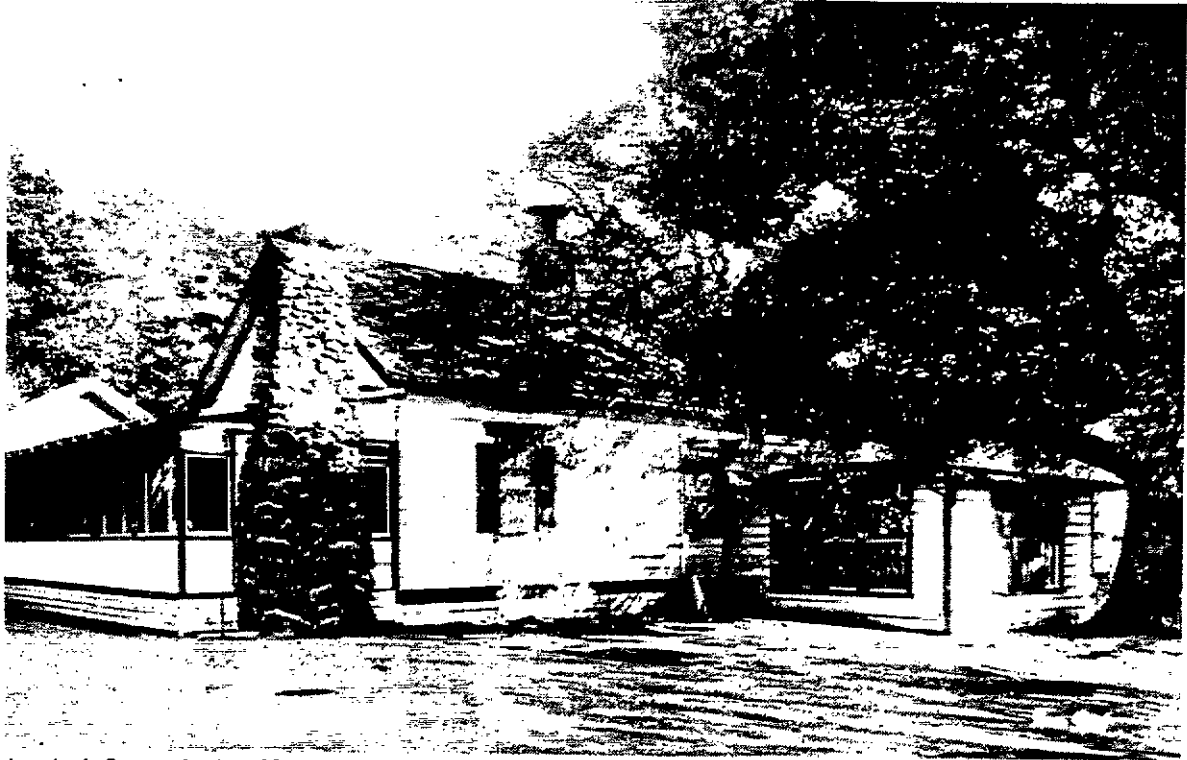
London's Cottage in the 1930s. In that decade the rear porch was widened and enclosed with windows and a fireplace was added. The department's goal is to remove these additions and return the cottage to a 1916 appearance.
