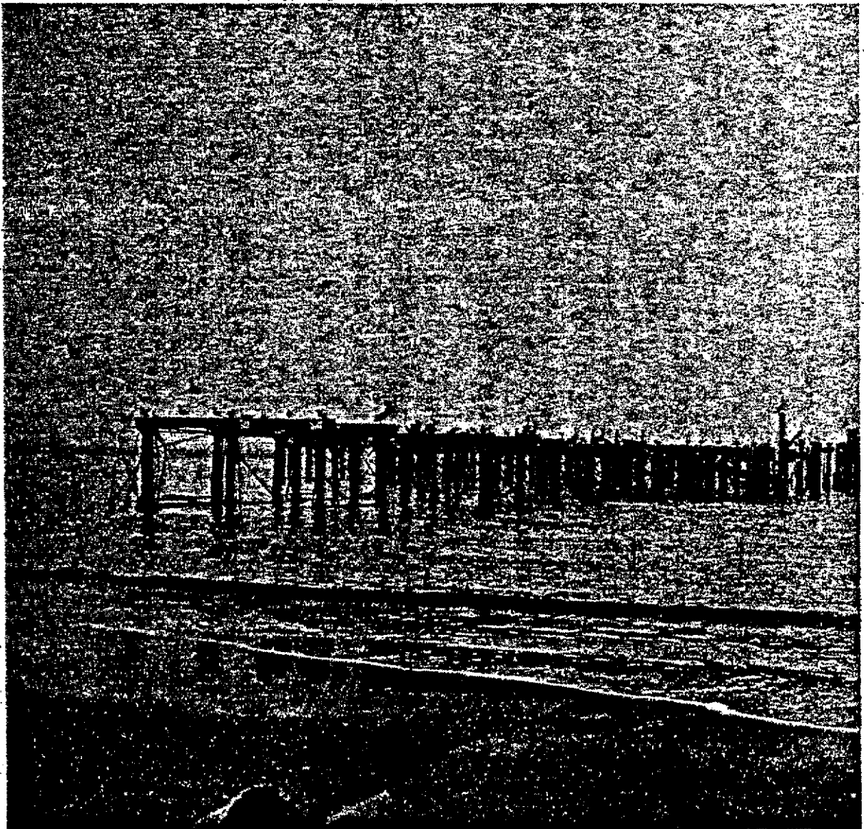
Remnants of West Garrison pier.
