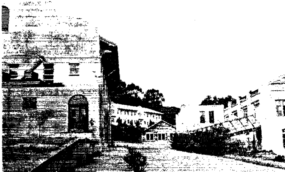
East Garrison buildings are in various stages of deterioration.
