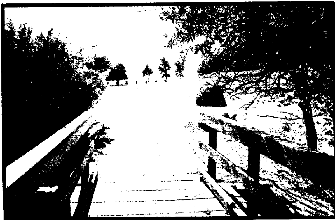
Bridge over Adobe Creek (1985)
