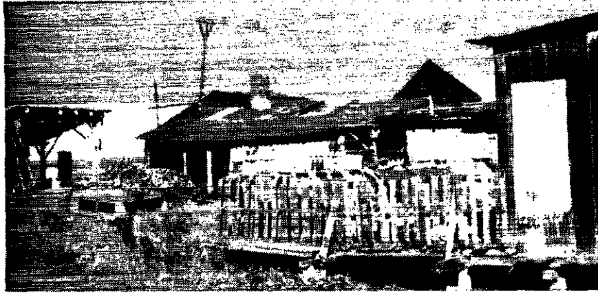
Buildings Nos. 6 and 8
