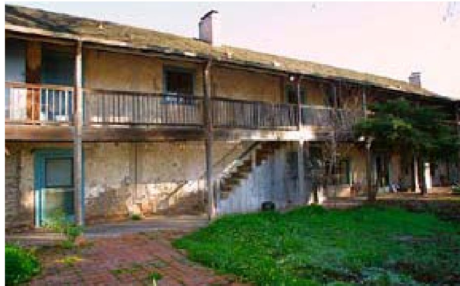
Photograph A: Blue Wing Inn, south elevation from courtyard, 2002.
