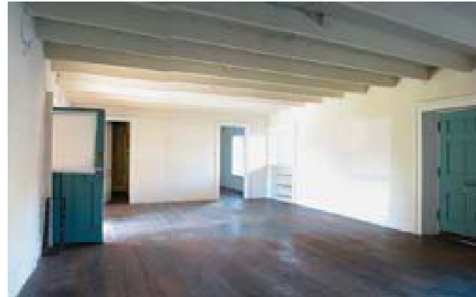
Photograph B: Blue Wing Inn, ground level interior, 2002.
