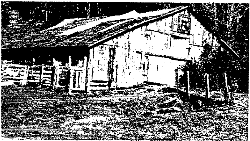
Barn near southeast shoreline of Stone Lagoon
