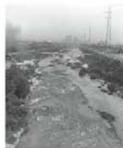
North of 7th at viaduct
