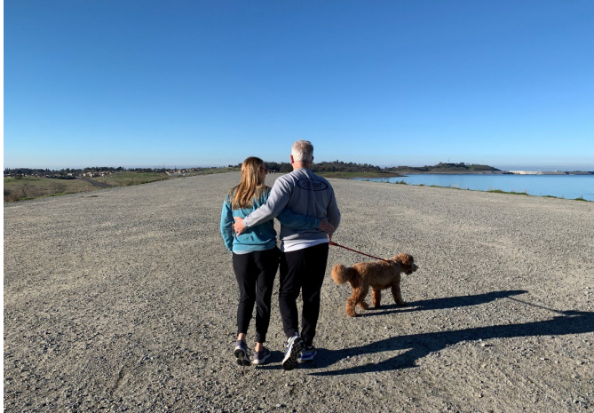
Pedestrians at Mormon Island Auxiliary Dam
