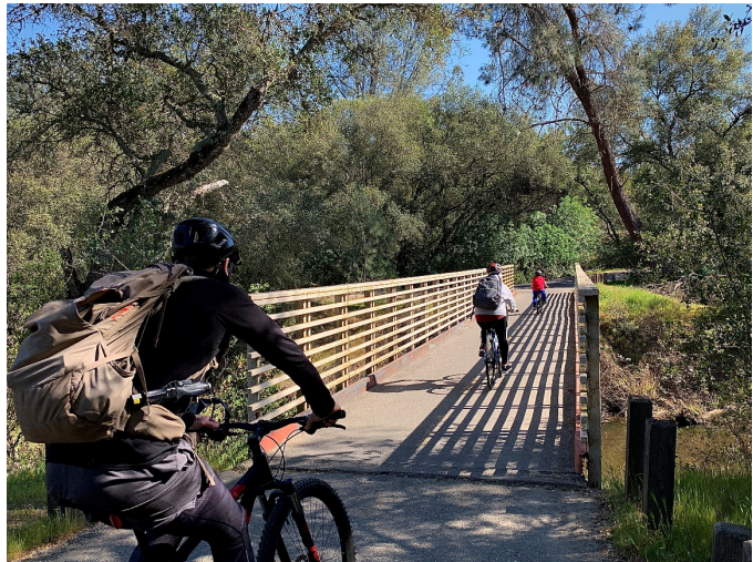
Willow Creek Bridge
