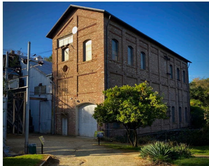
Folsom Powerhouse SHP, Main Powerhouse
