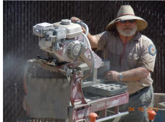
Leon Jordan cutting concrete blocks
