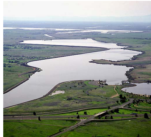
Thermalito Forebay (view southwest)
