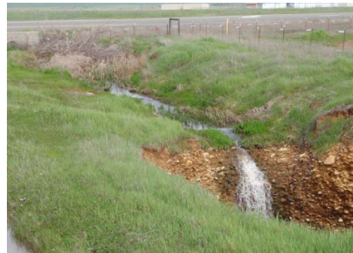
Drainage from north culvert under Larkin Rd.
