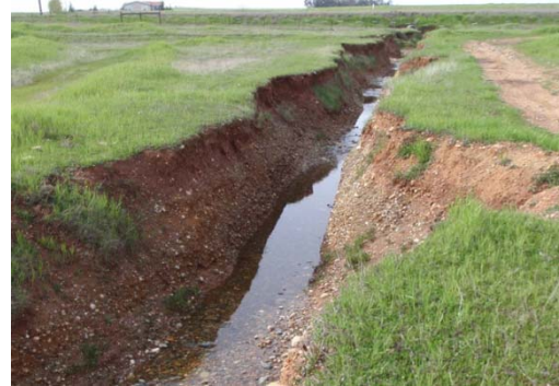
Drainage from southwest culvert under Larkin Rd.
