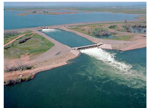
Thermalito Afterbay (view northwest)
