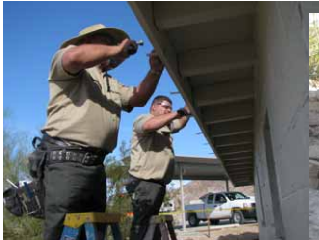
Leon Jordan and Marco Guzman are busy attaching rain gutters.
