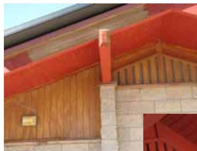
Fresh paint adorns the restroom building.
