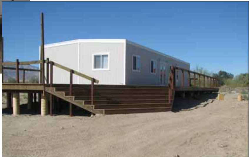
The Discovery Center now has a new deck and stairs.
