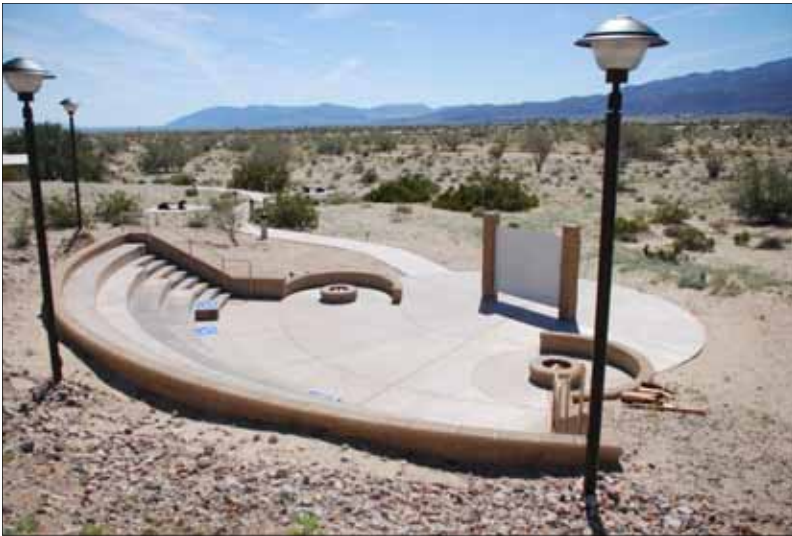
The new Ocotillo Wells amphitheater.
