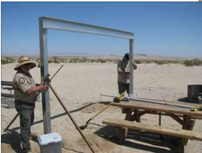
Leon and Jeff work on a metal shade structure.
