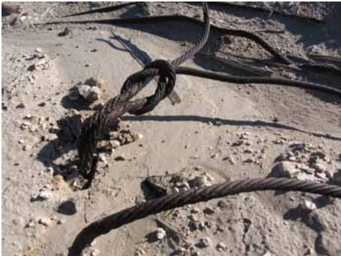
Cables that were used to hold down the oil derrick at the Routhe Well.
