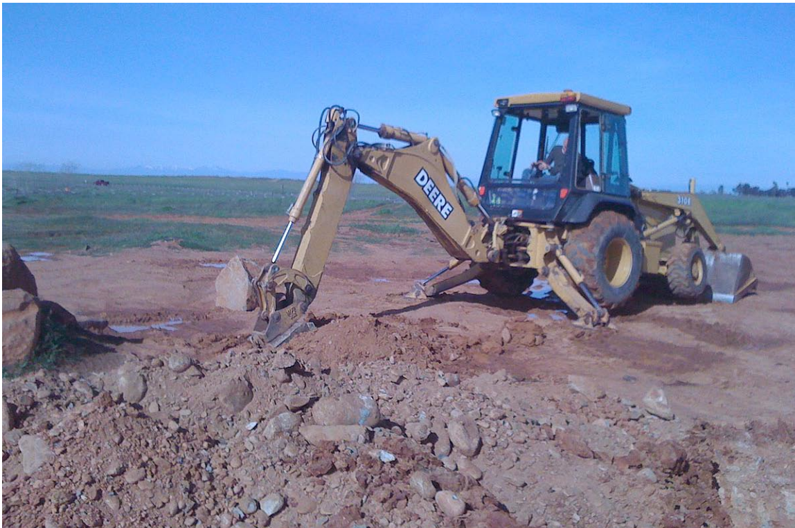
Photo No. 2 Excavated Laguna Formation
