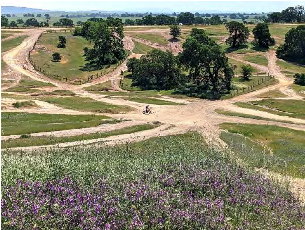
Prairie City SVRA includes varying topography, which is an important consideration for the design, construction, and maintenance of sustainable roads and routes.
