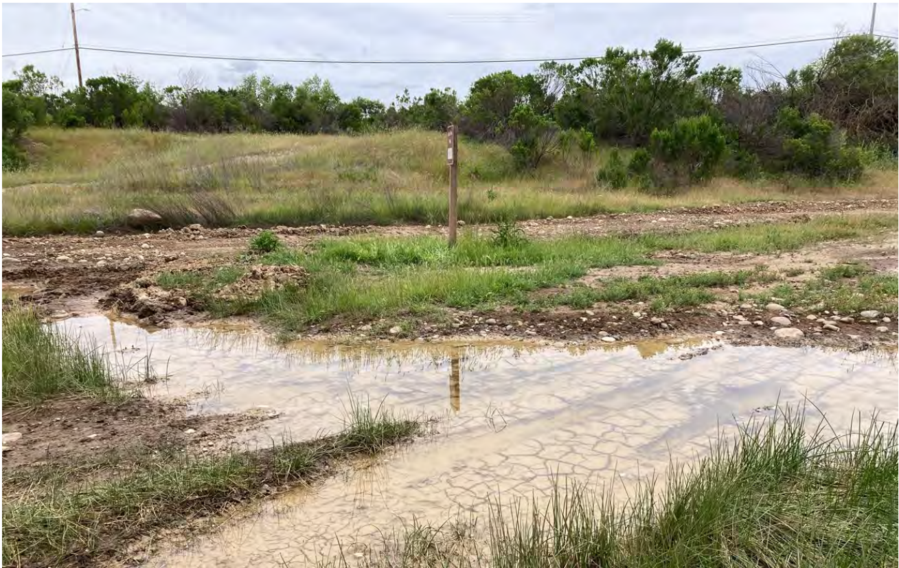
Although portions of Prairie City SVRA restrict OHV use due to existing water features or wetland areas, some routes intercept these features and can create erosion issues or alter the drainage patterns.
