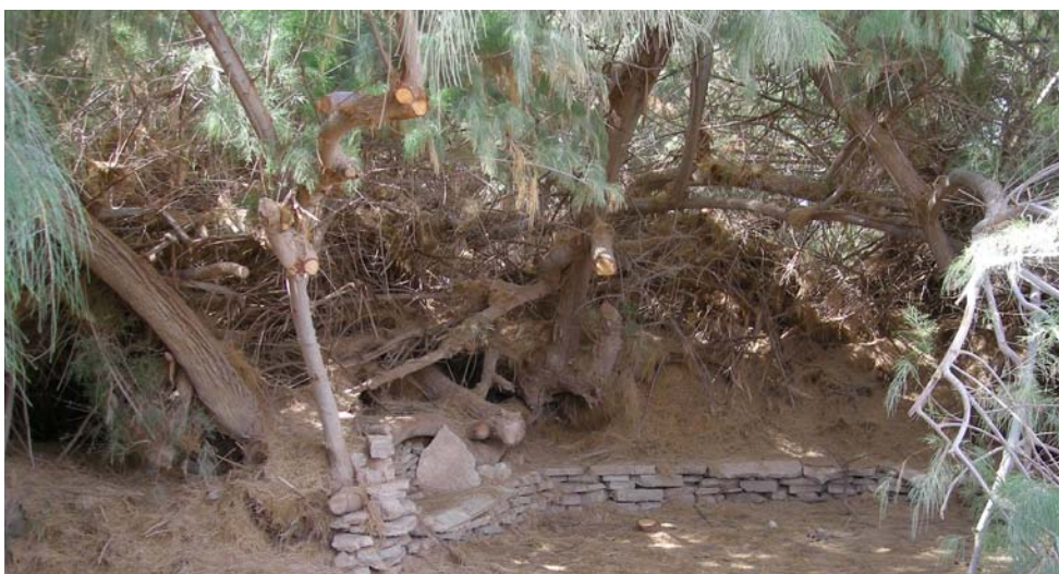
Stone retaining wall.
