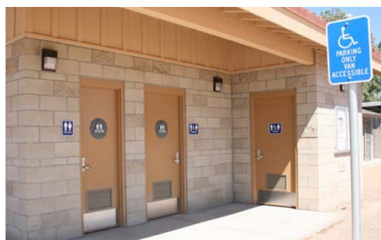
ADA accessible restroom facility.
