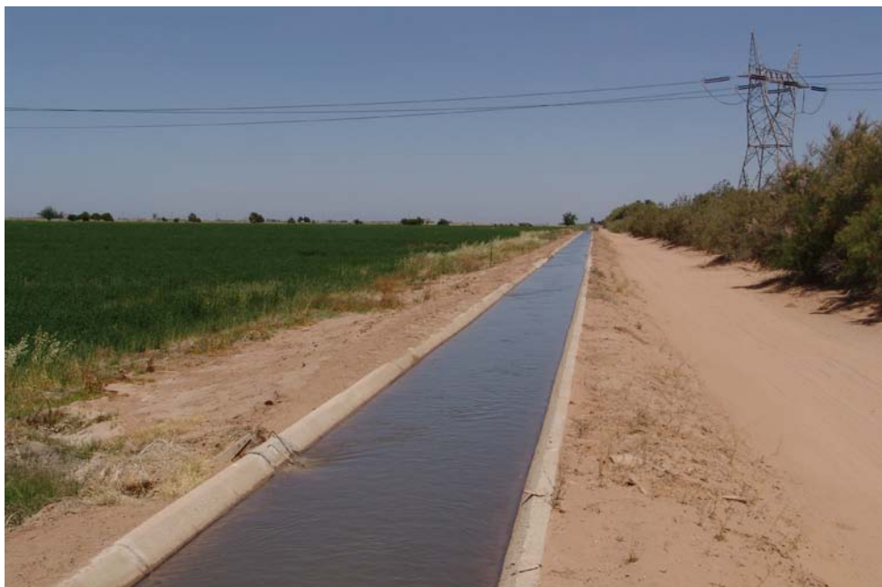
Adjacent agricultural land, South Alamo Canal, and perimeter road.
